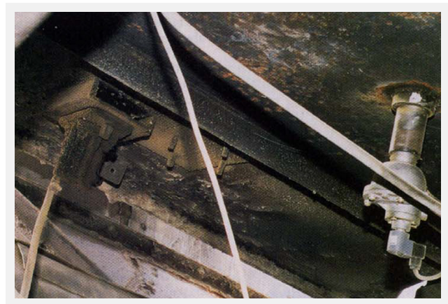
Past attempts to move fly ash with other equipment, such as the pneumatic vibrator shown on the left, proved ineffective. AirSweep unit is on the right.
